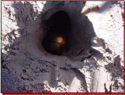
Exposed PVC Pipe Using Non-Destructive Excavation
