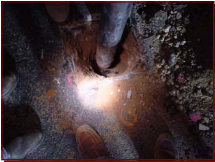
Non-Destructive Excavation During SUE Night Activity
