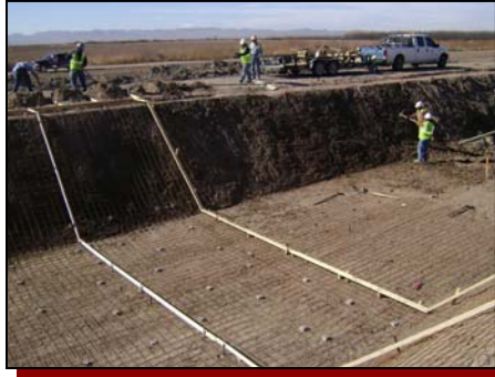
Phase 1A: Contractor is Setting Foundation for Concrete Riprap
